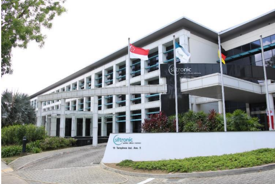
Siltronic's existing facility at JTC's Tampines Wafer Fab Park
